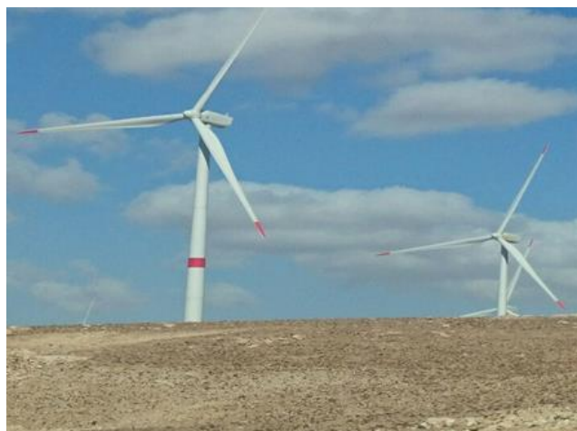
Figure 3. It is a Famous type of wind electric generators. (21)
